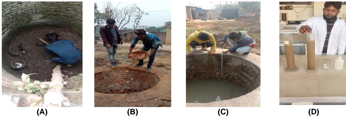
Picture 1. Drywell recharge work in selected sites of District Ambedkarnagar
