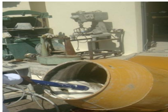
Fig. 2. Mixing procedure of the foamed concrete
