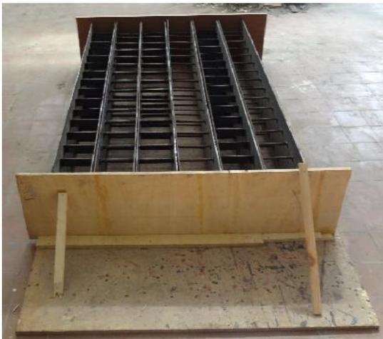
Fig. 4. Formwork in vertical position for concrete pouring
