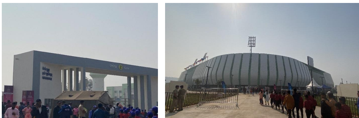
Fig. 5. Entry & Exit Gates with crowd management at Birsa Munda Stadium, Rourkela
